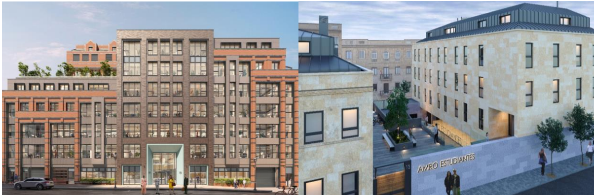
Refurbishment of a 7-Storey Green Office in Birmingham
